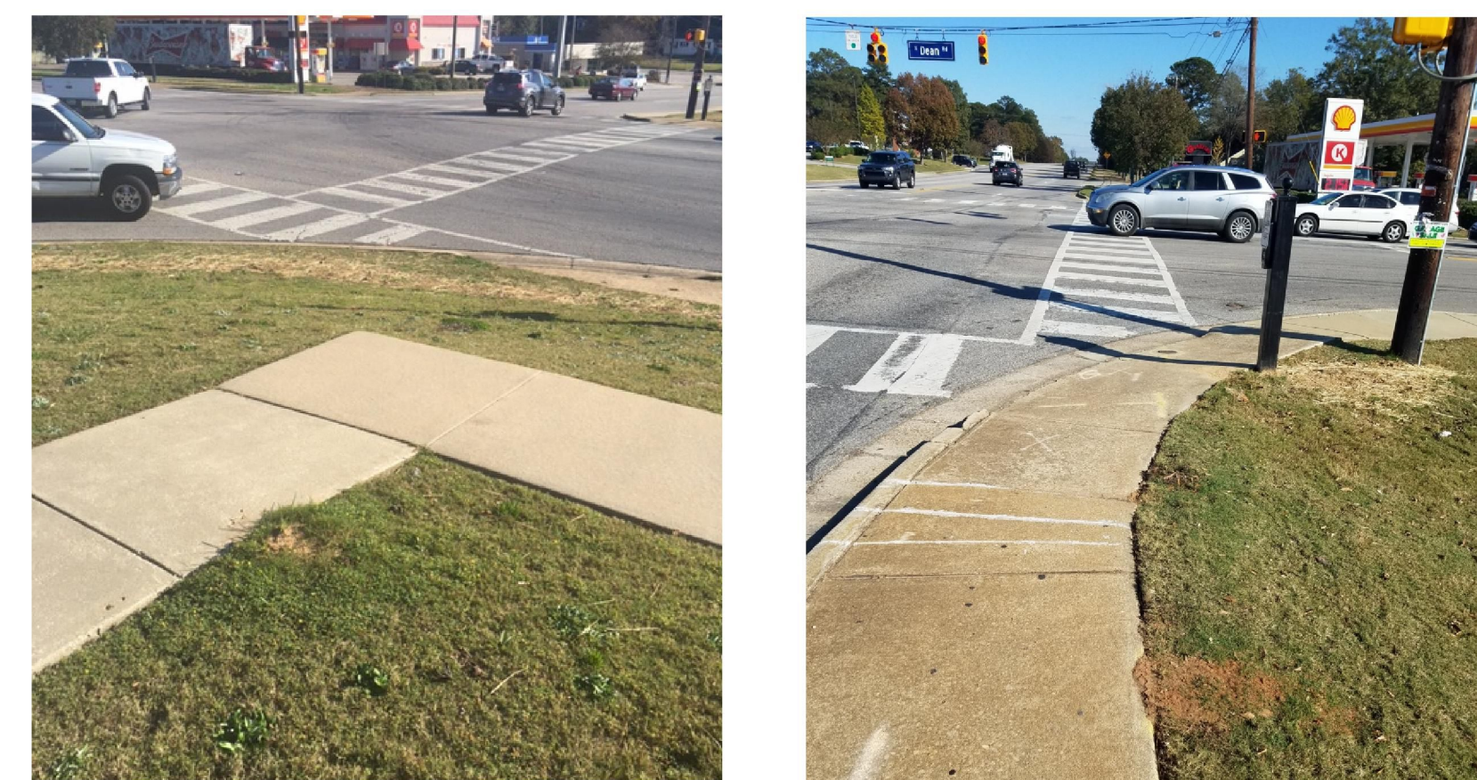
Poor sidewalk need to improve
